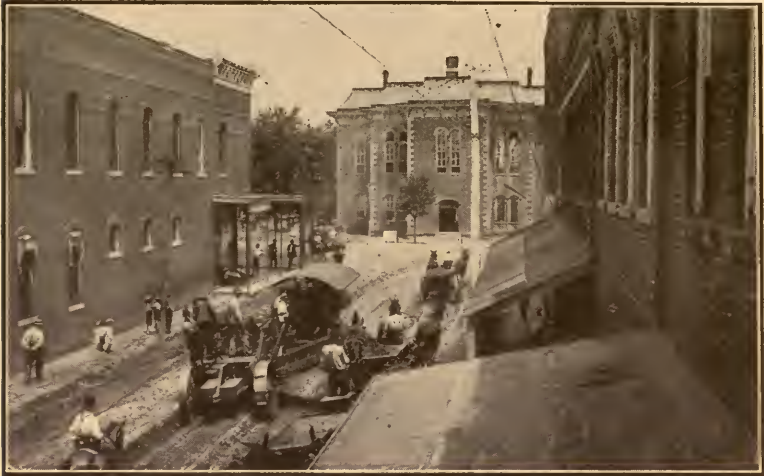
SOUTH MAIN STREET, BENTON (PAVING)
